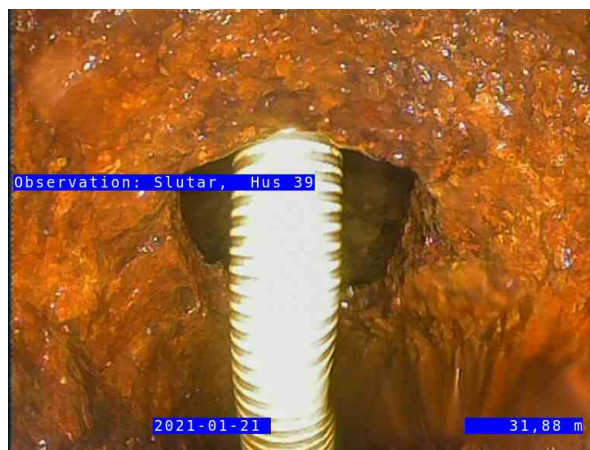
5_0001.jpeg, 00:00:02, 31.88m Slutar, Hus 39 / Hus 39
